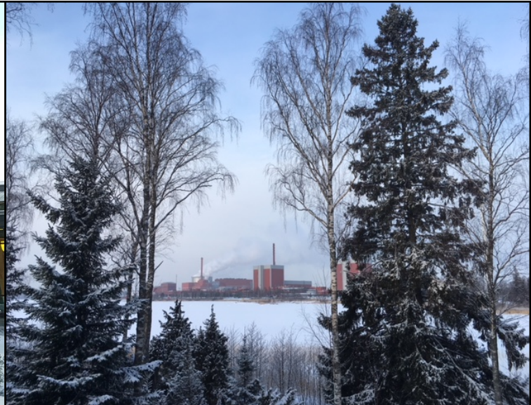
Olkiluoto Nuclear Power Plant
