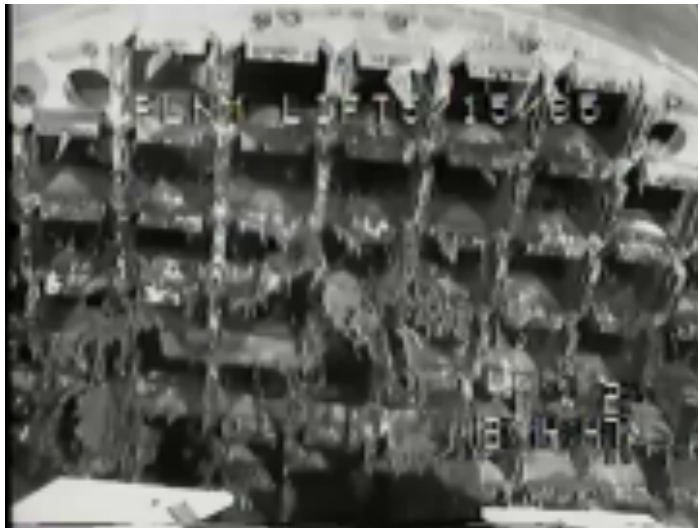
Bottom of the Upper Core Support Assembly
