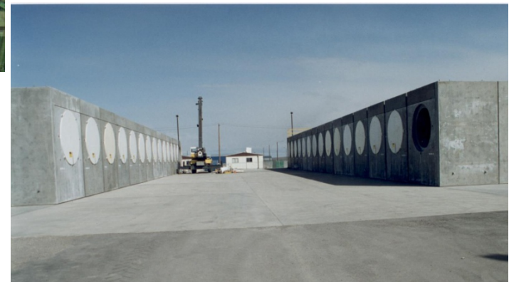
2000 – 2001 Removed from pool, dewatered, dried, and placed in dry storage
